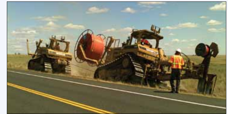
▲ NoaNet construction crew building out high-speed broadband fiber in Eastern Washington.
